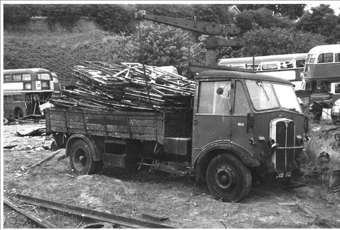
Photo 1938, by Bob Martin , added to LTSV on 07/06/2007. Photographed in a scrap-yard at Stratford upon Avon in about 1964, 95Q had served LT between 1936 and 1963. Based on an AEC Mercury chassis, it has the distinctive crane and bolster typical to pole carriers. Comment by Ray on 20/01/2010: There is a photograph of a pole carrier (in Loughton garage) in the LTM collection (1998/88201)
